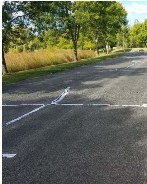
Figure 1. Road after sealing
