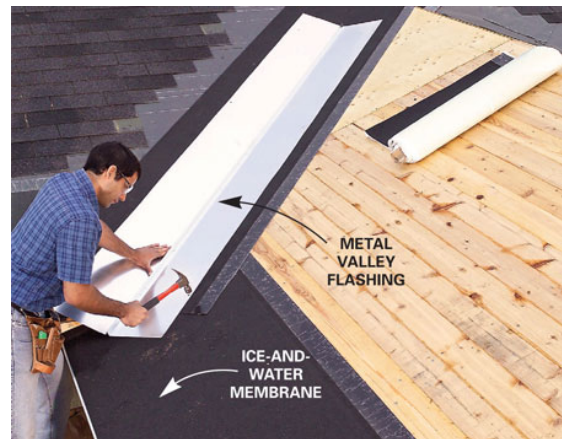
The installation of flashing in the new valley is shown. Note that existing shingles have been removed and ice and water barrier has been applied.
