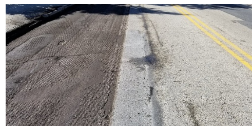
Figure 2 – Mill and overlay Streets
